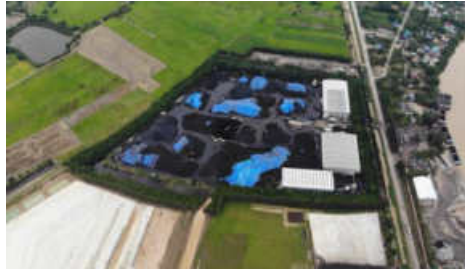
2. Stockpile and Screening Services
